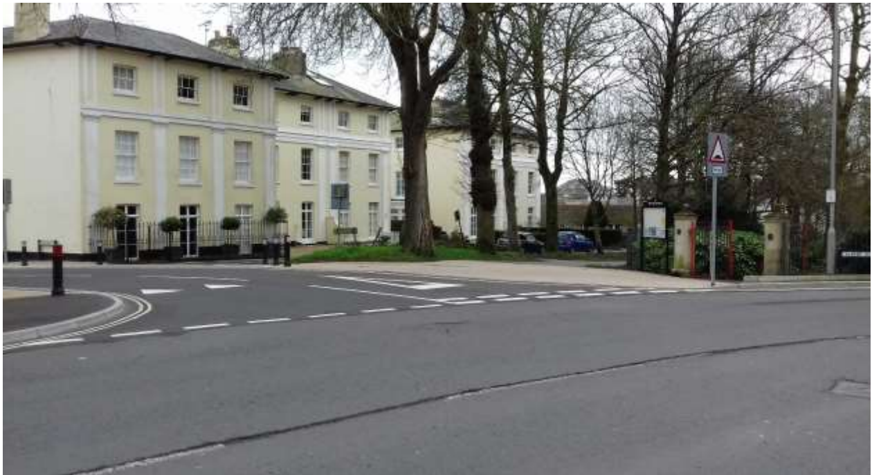
Junction after access improvement works, note wider footways, paved entrance, raised table and narrowed road width.
