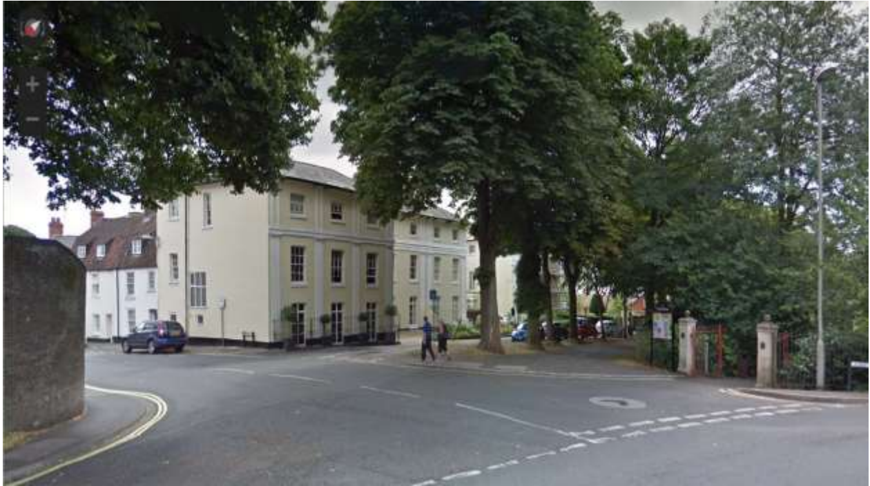
Junction Before works, main garden access gate bottom right.
