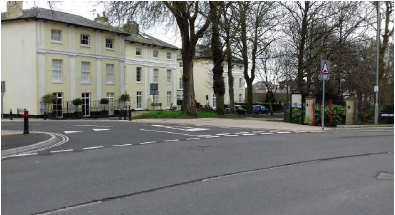
Junction after access improvement works, note wider footways, paved entrance, raised table and narrowed road width.
